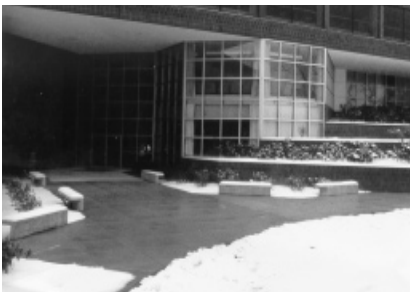
Figure 2.1B Office building (Digital)
