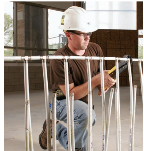
FostaPEX™ was chosen for the radiant tubing portion of the job because of its flexibility and form stability.
