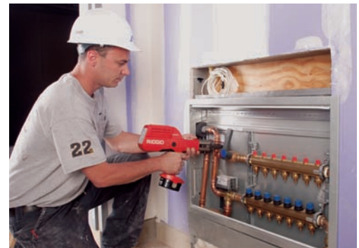
Kevin Bilo makes a ProPress connection at one of 11 Viega manifolds used to supply the 14,000-square-foot radiant heated space.
