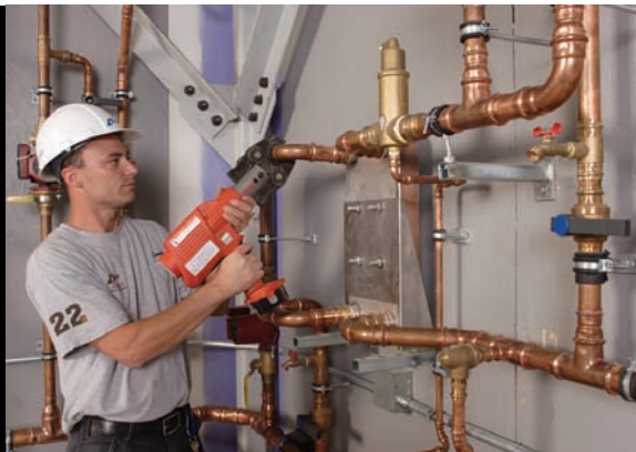
Kevin Bilo makes a ProPress connection at one of 11 Viega manifolds used to supply the 14,000-square-foot radiant heated space.
